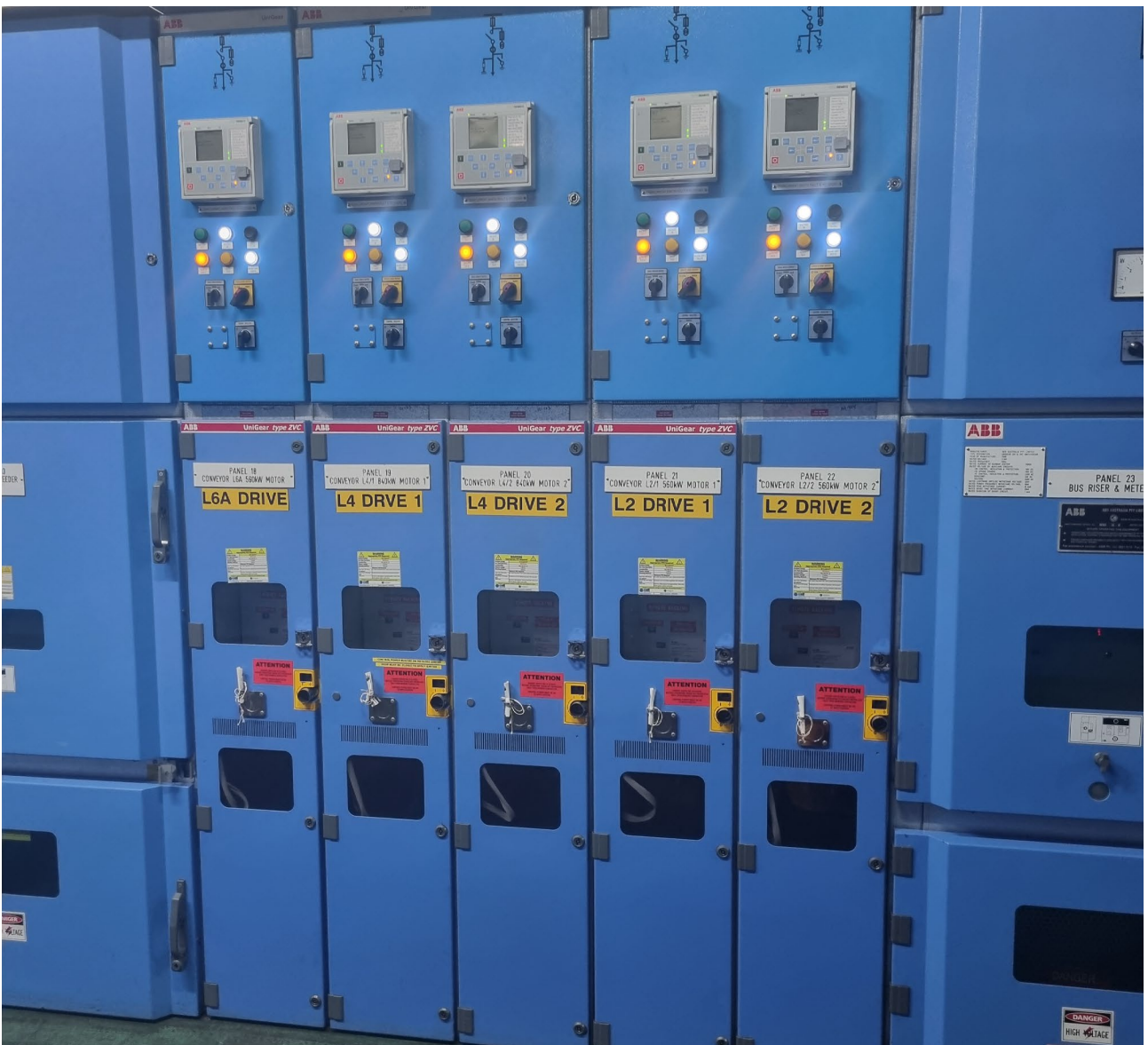
Figure 5 – New remote racking system complete and in operation
