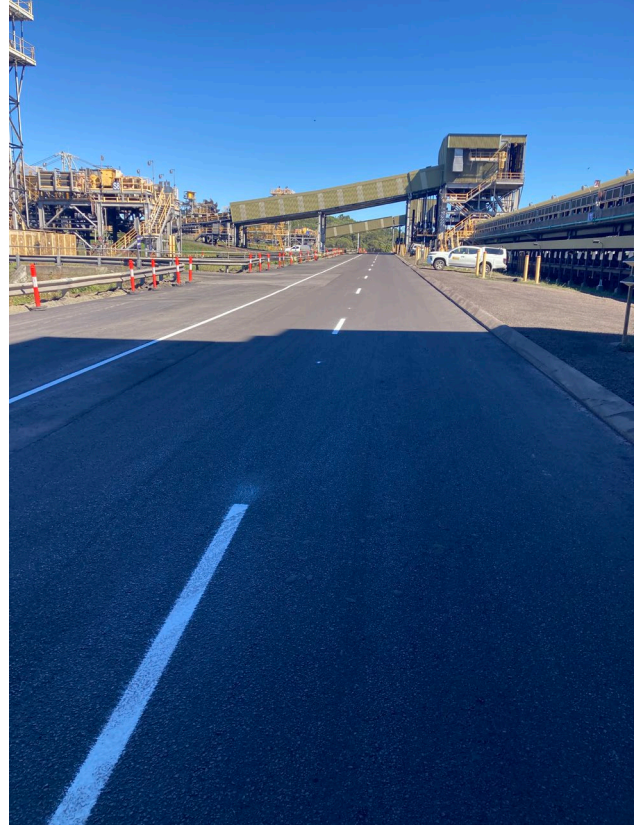
L1 southern lane (after). Resurfaced
