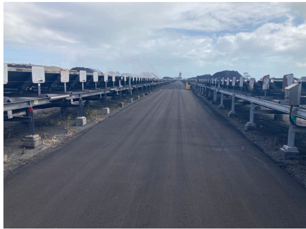
Bund 4 road, after reconstruction and resurfacing
