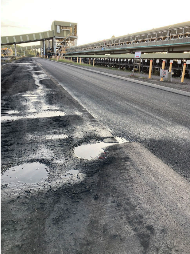
L1 southern lane (before). Typical surface condition
