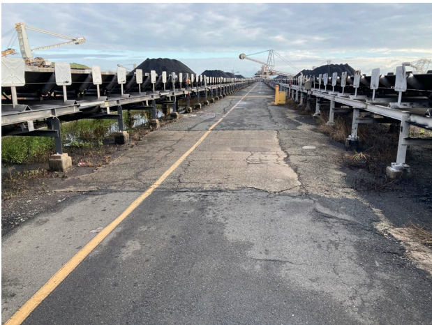
Bund 4 road (before). Typical surface condition
