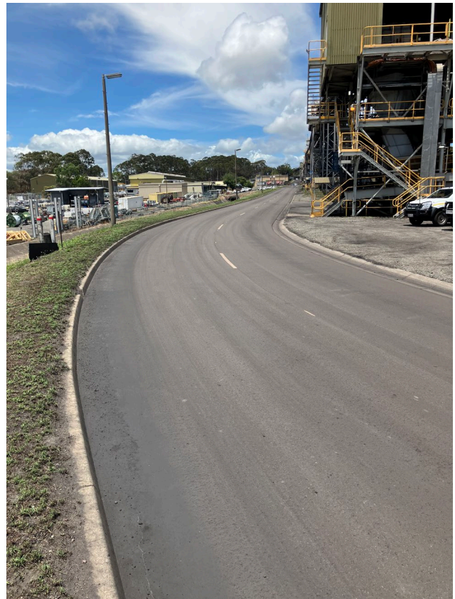
S4 road (after). Resurfaced
