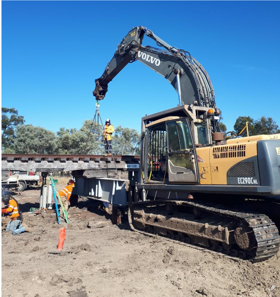
Figure 3-7 Replacement of substructure without impacting superstructure
