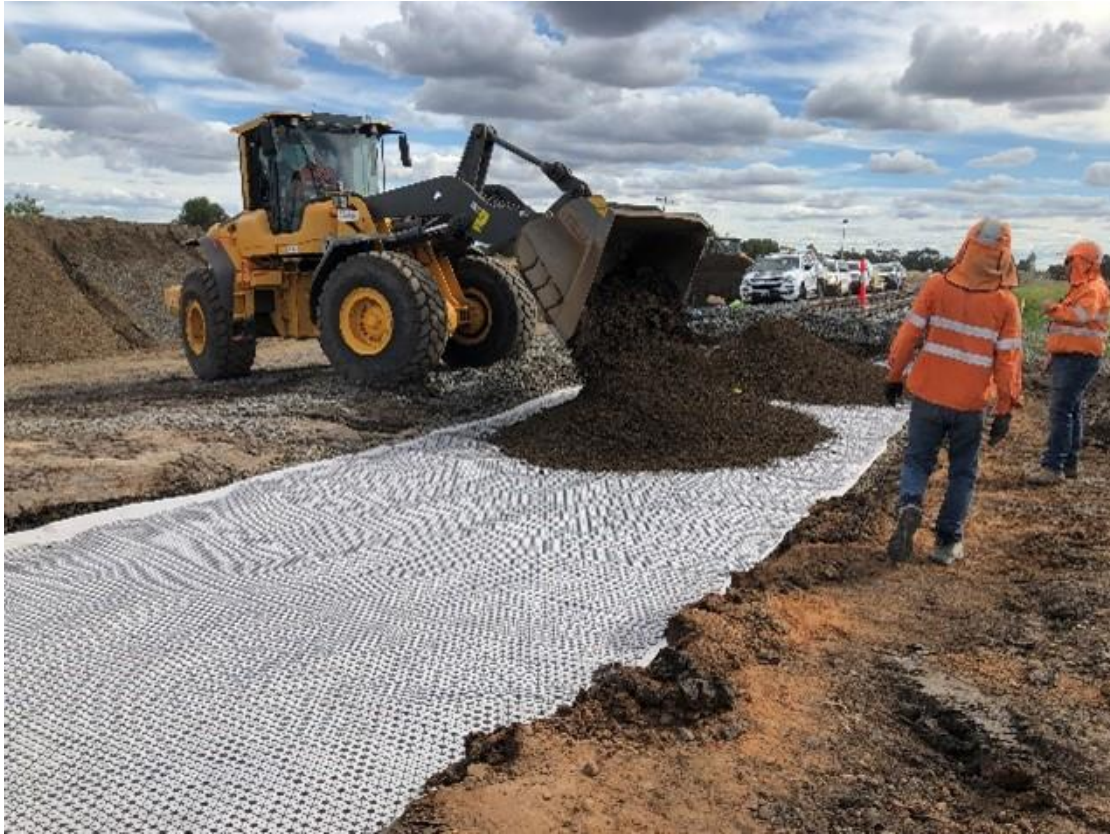
Figure 3-6 Previous formation strengthening works
